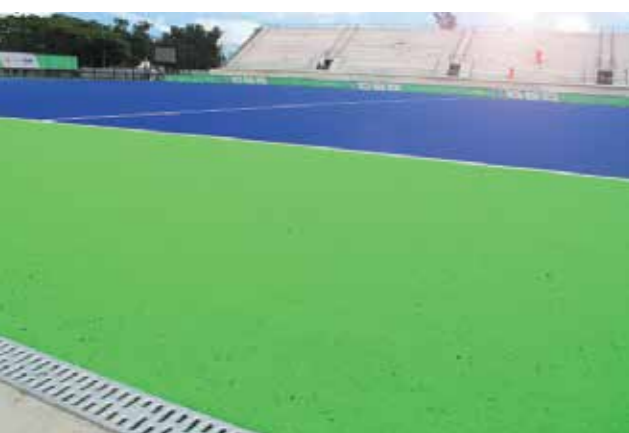
The hockey facility of the Olympic Games 2016 in Rio is equipped with ACO drainage channels
